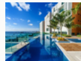
Cloc Marina Residence. Historic coastal restoration
